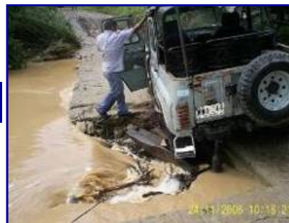
El Neme Creek bridge rebuilding
